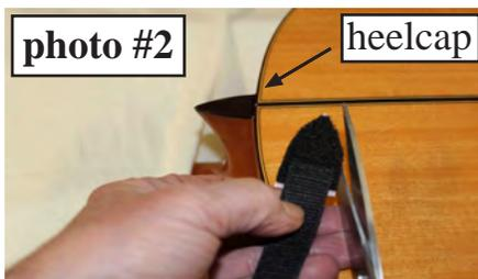
**Photo #2** - use scissors to trim the velcro loop of the attachment to match the outline of the heelcap
